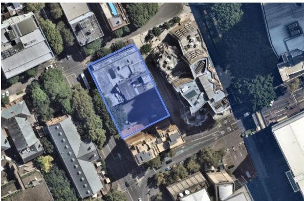
Figure 6: aerial, 622-644A Harris Street
