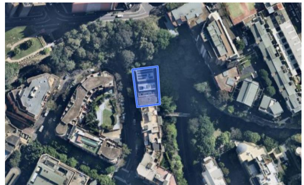
Figure 31: aerial, 14A Quarry Master Drive
